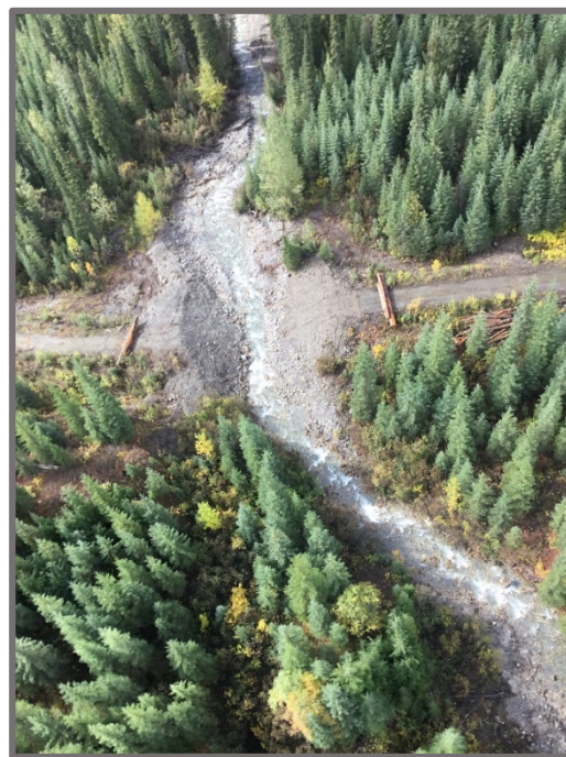
Road crossing of Tea Creek after Cooper Creek removed the bridge.
